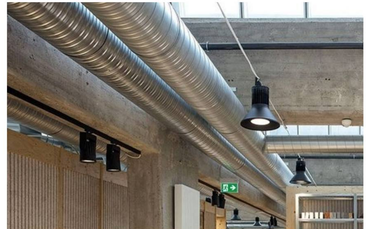
Figure 7.7: Thermaduct Thermaround Architectural Duct System
