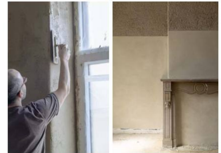
Figure 5.4-5: Clay Plaster
